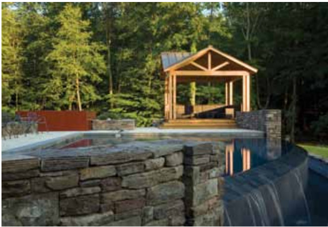
Stone walls with piers bordering negative edge
