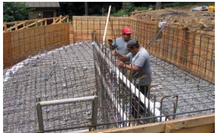
Reinforcing steel of main pool with interior dividing wall
