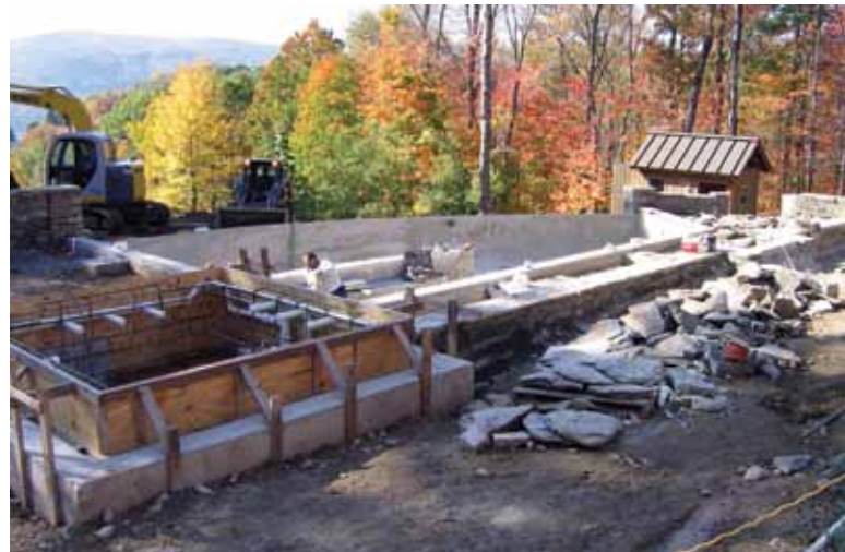
Walls formed for raised perimeter overflow spa
